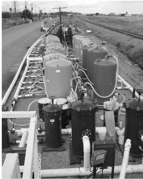
There are 30 media vessels containing 120,000 pounds of an organoclay/anthracite blend.
